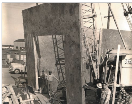
Andersen gets its start with Tilt Up Concrete
