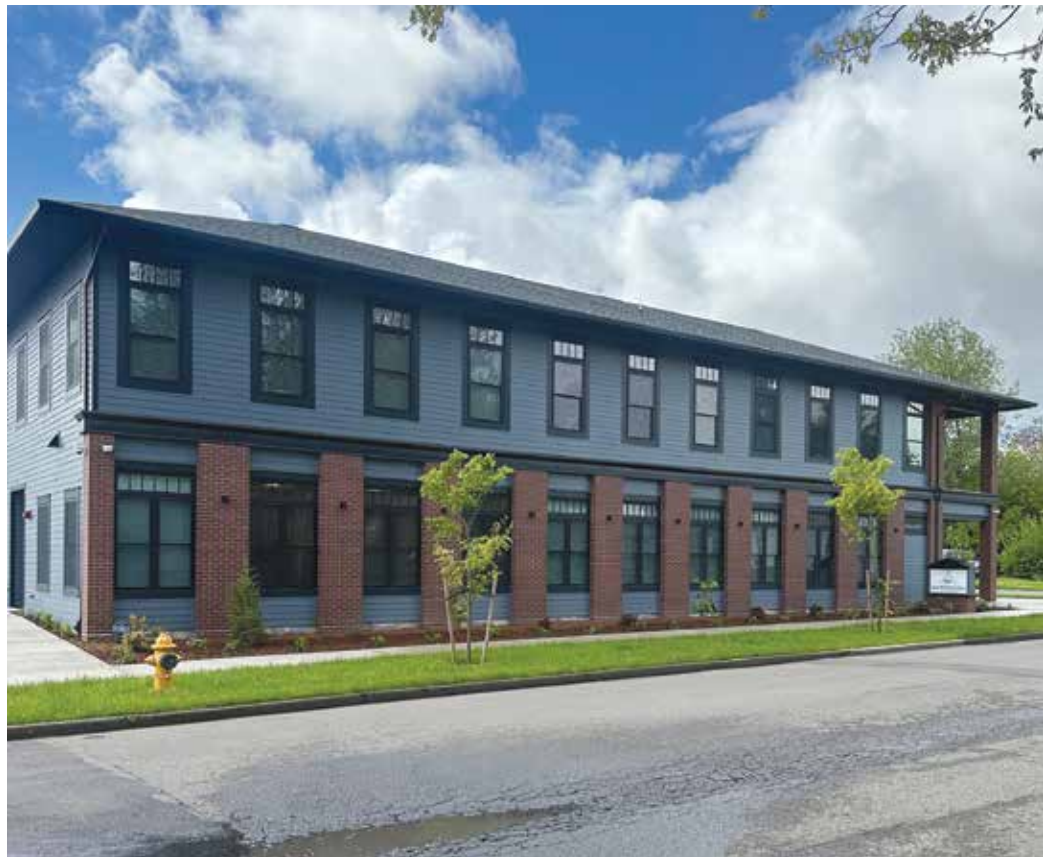
The new building is a wood-framed structure with exterior architectural elements, such as brick finishes and a metal wrapped cornice acting as an accent band around the building.
